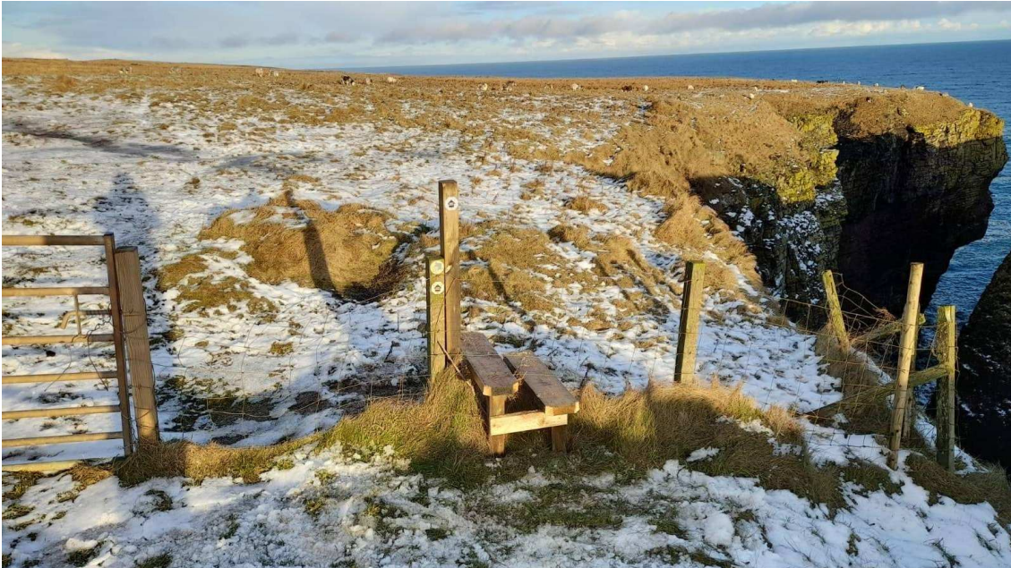
Above: One of the three new stiles at Corbigoe ( Stage 12 )
